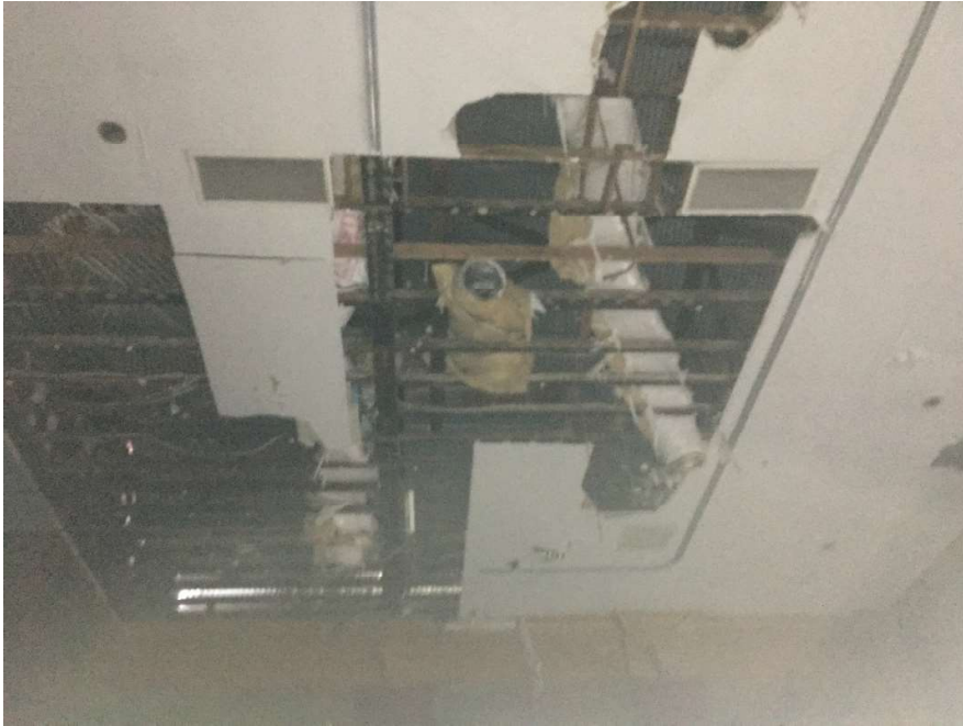
Photograph 7: Internal ceiling damage on second floor in main theatre area.
